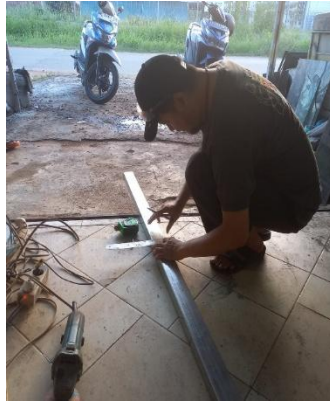
Gambar 3. 37 Proses Pengukuran Material Hollow
